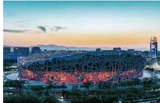
National Stadium Bird's Nest Project
